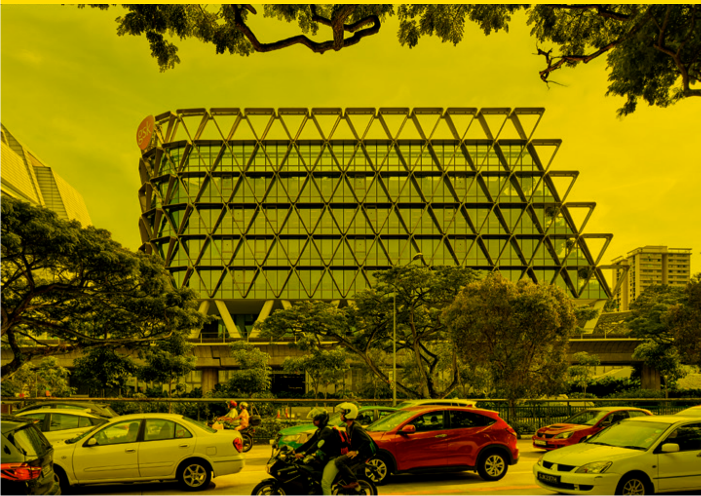
The GSK Building has an elaborate curtain wall system that includes an elaborate triangular-patterned brise-soleil system. On the top floor, this brise-soleil system breaks away from the glazing to become its own filigree silhouette.
